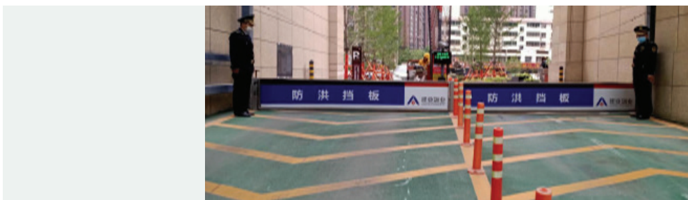
FLOOD CONTROL BAFFLES AT BASEMENT ENTRANCE IN THE COMMUNITY
