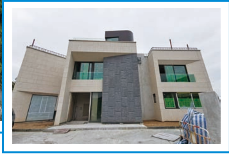
Tai Mong Tsai, Sai Kung, N.T., Hong Kong (Lot 243 S.A. in DD 252) Superstructure Works Main contractor for one residential house including E&M works
