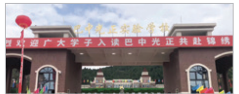
Bazhong Guangzheng Preparatory School
