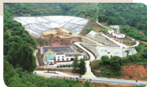
Nanyang collection and landfill project
