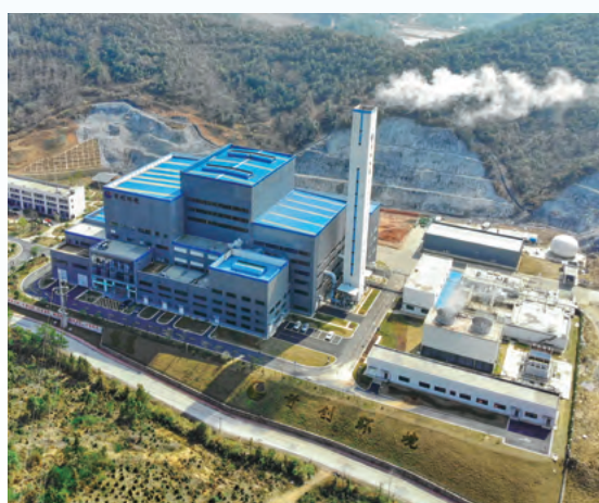
Gao'an Power Plant
