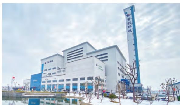
CEHL’s new waste incineration project in Sui County of Henan Province was a project-in-reserve during the year and plans to enter operations in 2020
