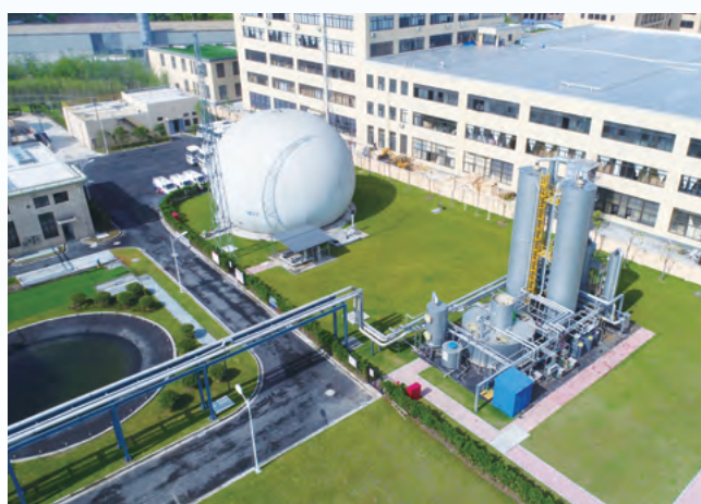
Hangzhou Anaerobic Treatment Project
