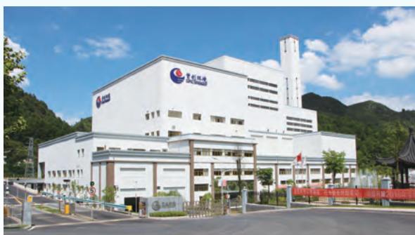
Duyun Power Plant
