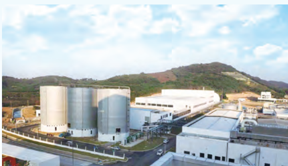
Ningbo Anaerobic Treatment Project
