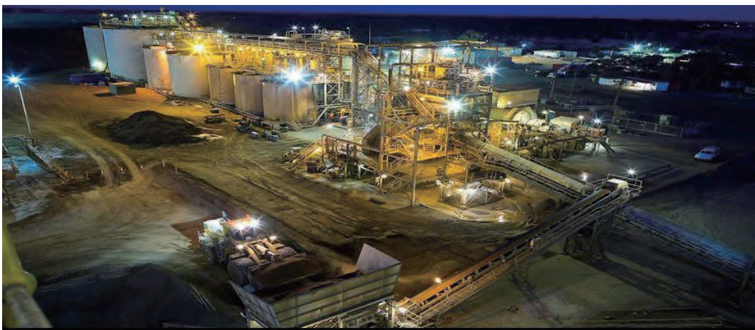
Figure 47: The Marvel Loch Processing Facility (2)
