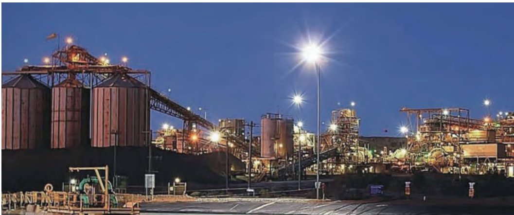
Figure 46: The Marvel Loch Processing Facility (1)
