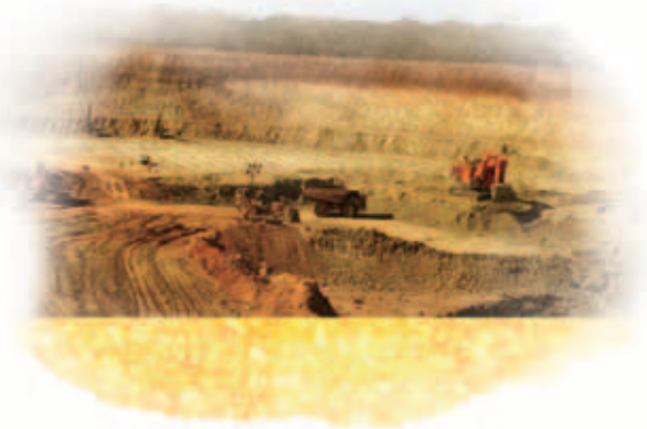
Cornishman South Open Pit of the Australia Gold Project
