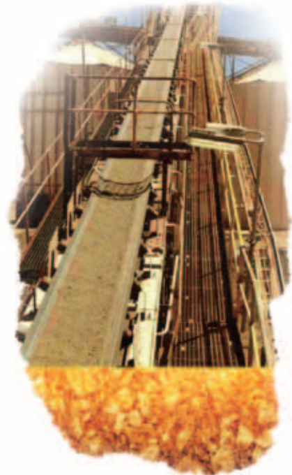
Dry commissioning of the processing plant commenced on 18 December 2014
