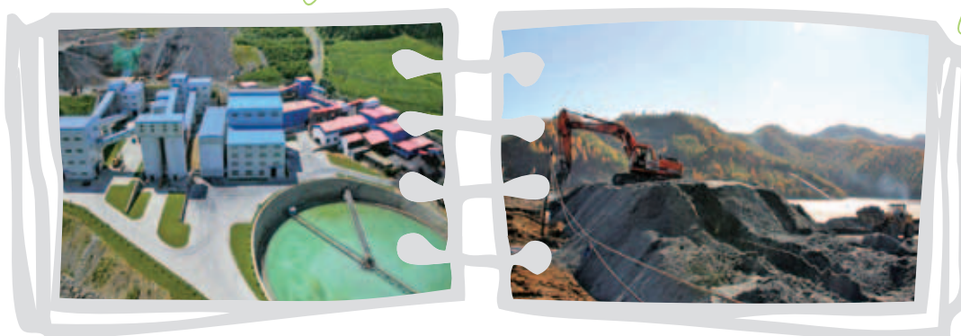
Lower right corner of the picture below is the thickening pool of the tailing pulp concentration and overflow water recycling system of Aoni Mine
