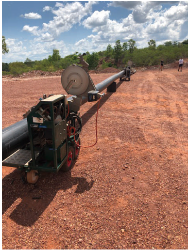
Figure 5: Dewatering pipeline being setup at the flagship Rustlers Roost open-pit
