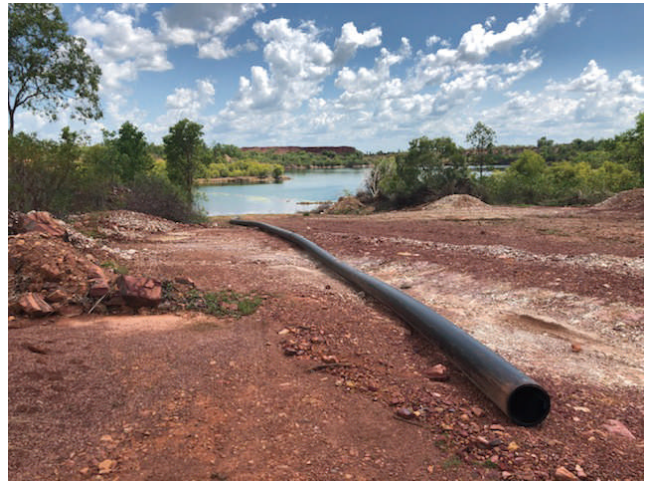
Figure 5: Dewatering pipeline being setup at the flagship Rustlers Roost open-pit
