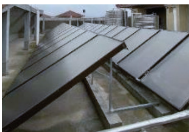
Solar water heating system
