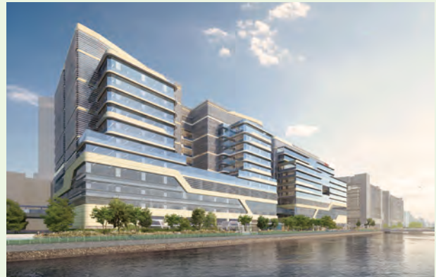
New Acute Hospital at Kai Tak Development Area (Site B)
