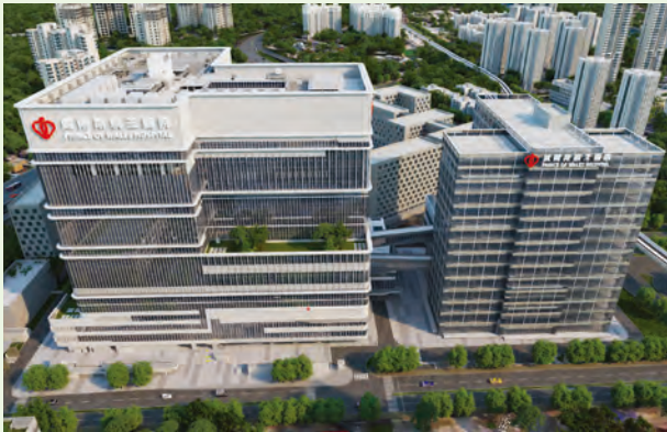
Main Works for In-Patient Extension Block for Redevelopment of Prince of Wales Hospital Phase 2 (Stage 1)
