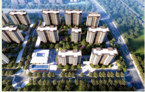
Government Targeted Repurchase Project (Plot 3), Fengdong New Town, Xixian New District, Xi'an, Shaanxi Province
