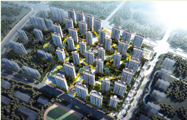
Siyi Real Estate Hushan Family Project, Tianjia'an District, Huainan, Anhui Province
