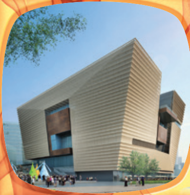
Construction of The Hong Kong Palace Museum
