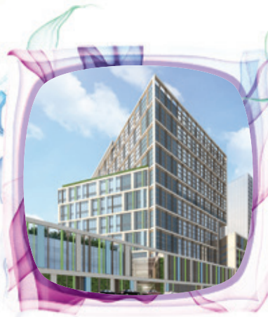
Construction of Redevelopment of Kwong Wah Hospital (Phase 1)
