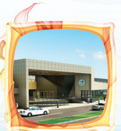
C340B-Main Works for Barra Station, Macao LRT
