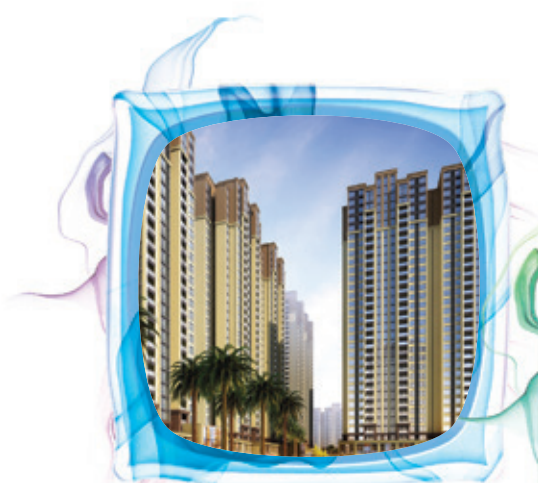
The Hongyong Garden Relocation Housing Project, Chengdu, Sichuan Province
