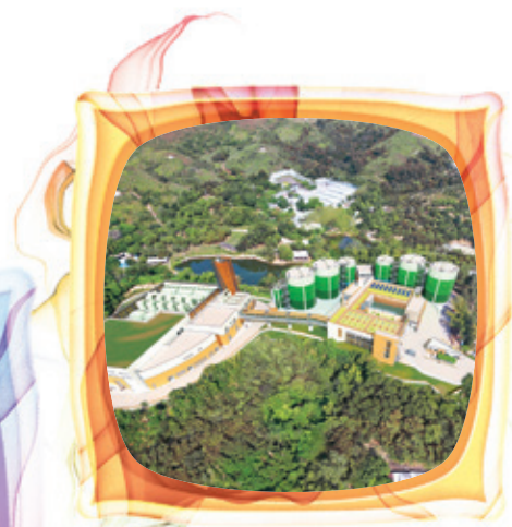
Organic Waste Treatment Facilities Phase 2
