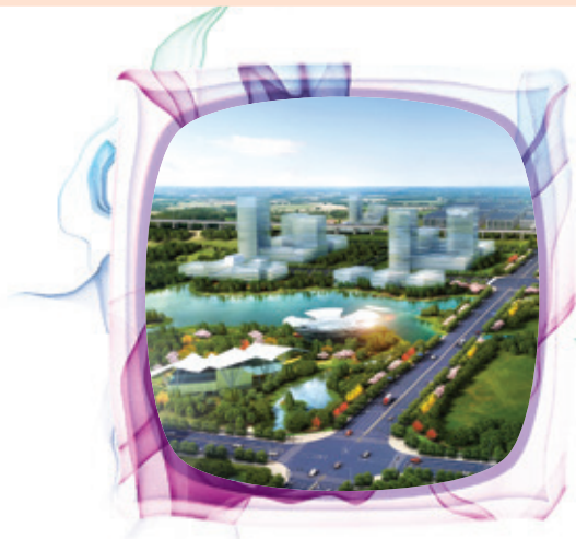
Infrastructure of High-speed Railway New Town PPP Project, Huzhou, Zhejiang Province
