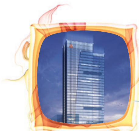
CSCI Engineering Headquarter Project, Hefei, Anhui Province
