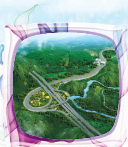
Leishan-Rongjiang Expressway PPP Project, Qiandongnan, Guizhou Province
