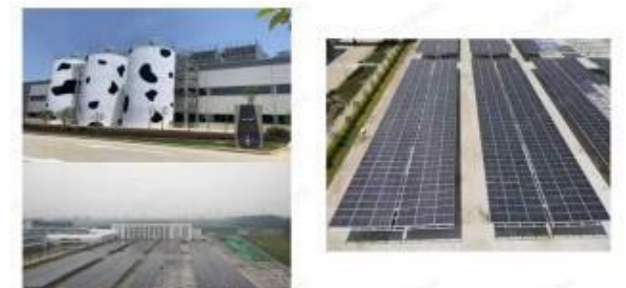
power generation of photovoltaic panel in Mengniu's factory in Wuhan
