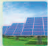
Solar Energy Solution
