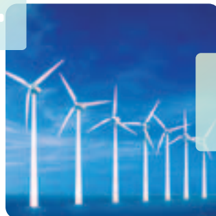
Wind Power Automation Control Solution
