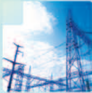
Power Remote Monitoring Solution
