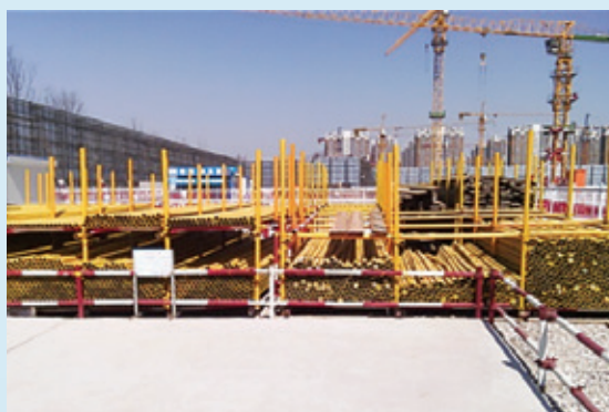
Material stacking rack
