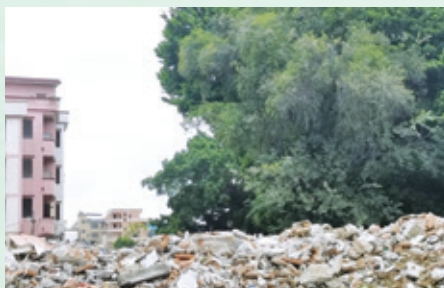
An ancient tree standing intact at the demolition site
