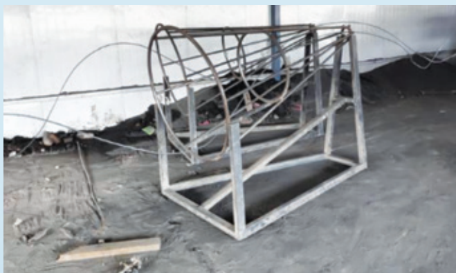
Protection for rebar straightening
