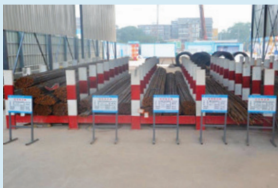
Rebar stacking rack
