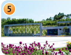
5 China Scivest WTE plant (Phase 2) (Undergoing preparatory works)
