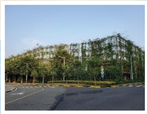
Landscaping to increase greenery coverage in our WTE plants
