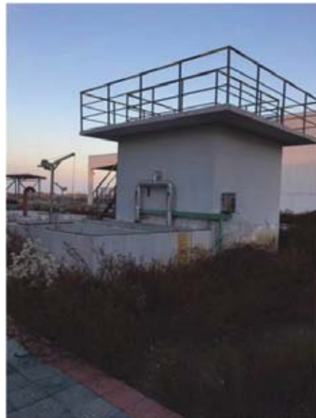
Sewage Station — Sludge Tank
