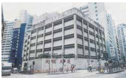
105-113 Ta Chuen Ping Street, Kwai Chung
