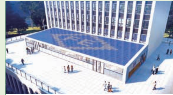
BIPV Reconstruction Design of the Second Floor of Far East (Zhuhai) Canteen
