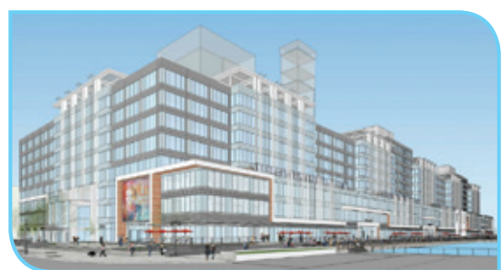
Harbourside Phase 1 & 1A, New Jersey, USA
