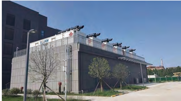
China Unicom Northwest Intelligent Cloud Data Centre
