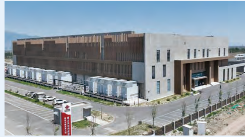
China Unicom (Huailai) Big Data Innovation Industrial Park
