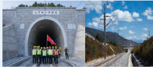
Cracking network coverage difficulties with leading technologies
