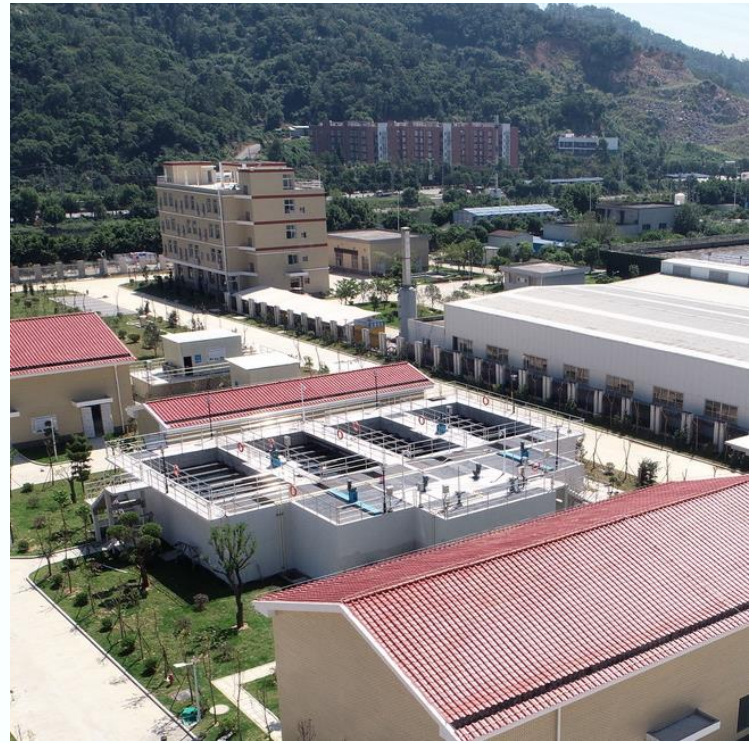
Our sewage treatment plant in Changle District, Fuzhou
