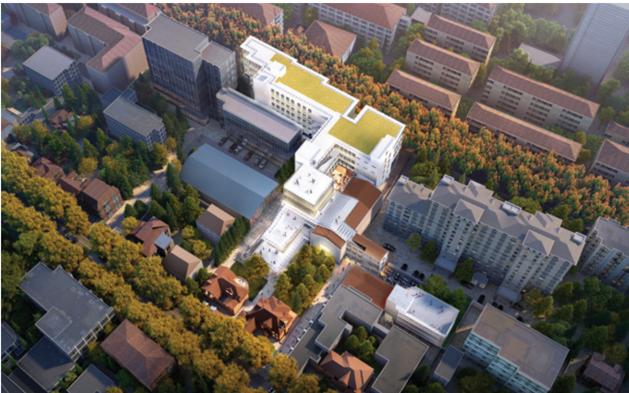
Wuyi Road project, Shanghai
