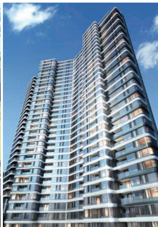
Site G89, Jiangning District, Nanjing
