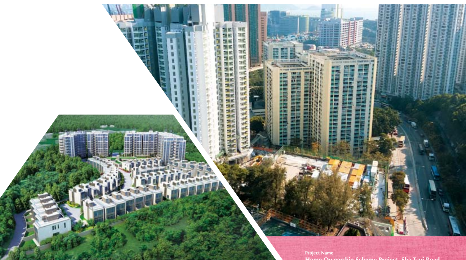
Project Name Residential Project, TMTL 427, So Kwun Wat Road, Tuen Mun, Hong Kong
